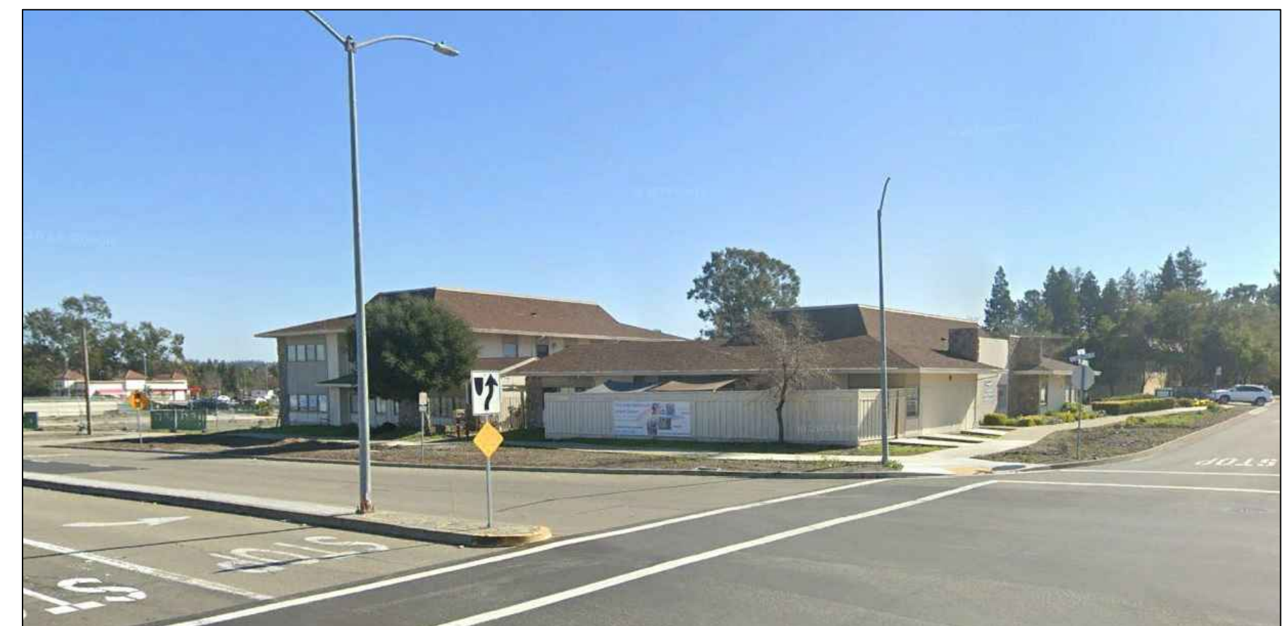
VIEW LOOKING SOUTHEAST ON DEERWOOD DR. 001
